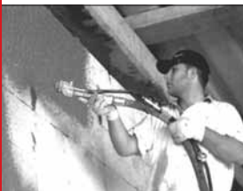
Premixed or traditional plasters spraying
