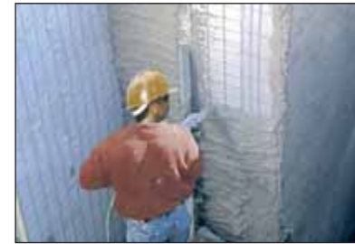
Mortar spraying on polystyrene panels with wire welded meshes
