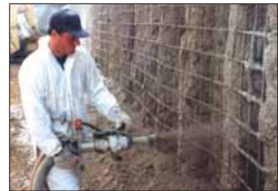
Spraying concrete
