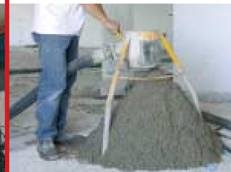
The floor screed conveyed at the upper floors
